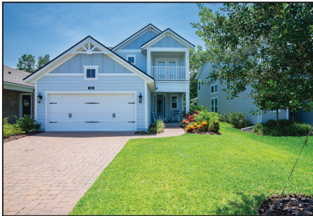
The home at 262 Pioneer Way Drive.
