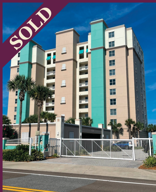
OCEANFRONT OCEANIA CONDOMINIUM UNIT 602 2 BEDROOMS | 2 BATH 1,325 SQUARE FEET
